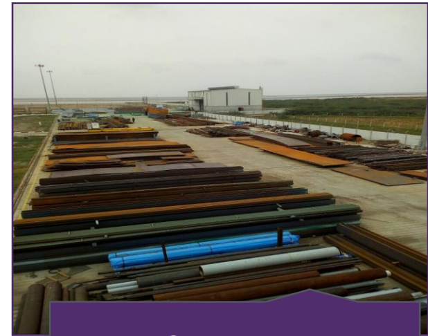
Material Storage Yard 30 M X 165 M
