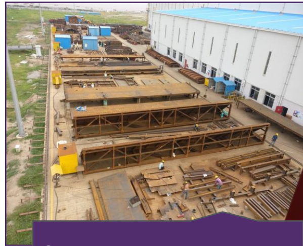
Open Fabrication Yard 25 M X 165 M
